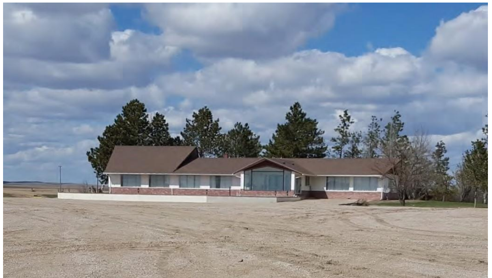
House at headquarters
